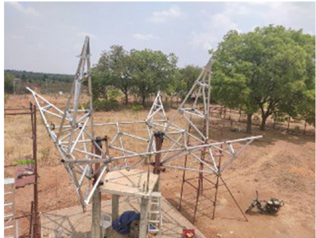
Figure 4. (Left) A view of the ELI telescope backup structure (right) Another view. Note the structure includes the assembled backup space frame for both the primary and secondary.
