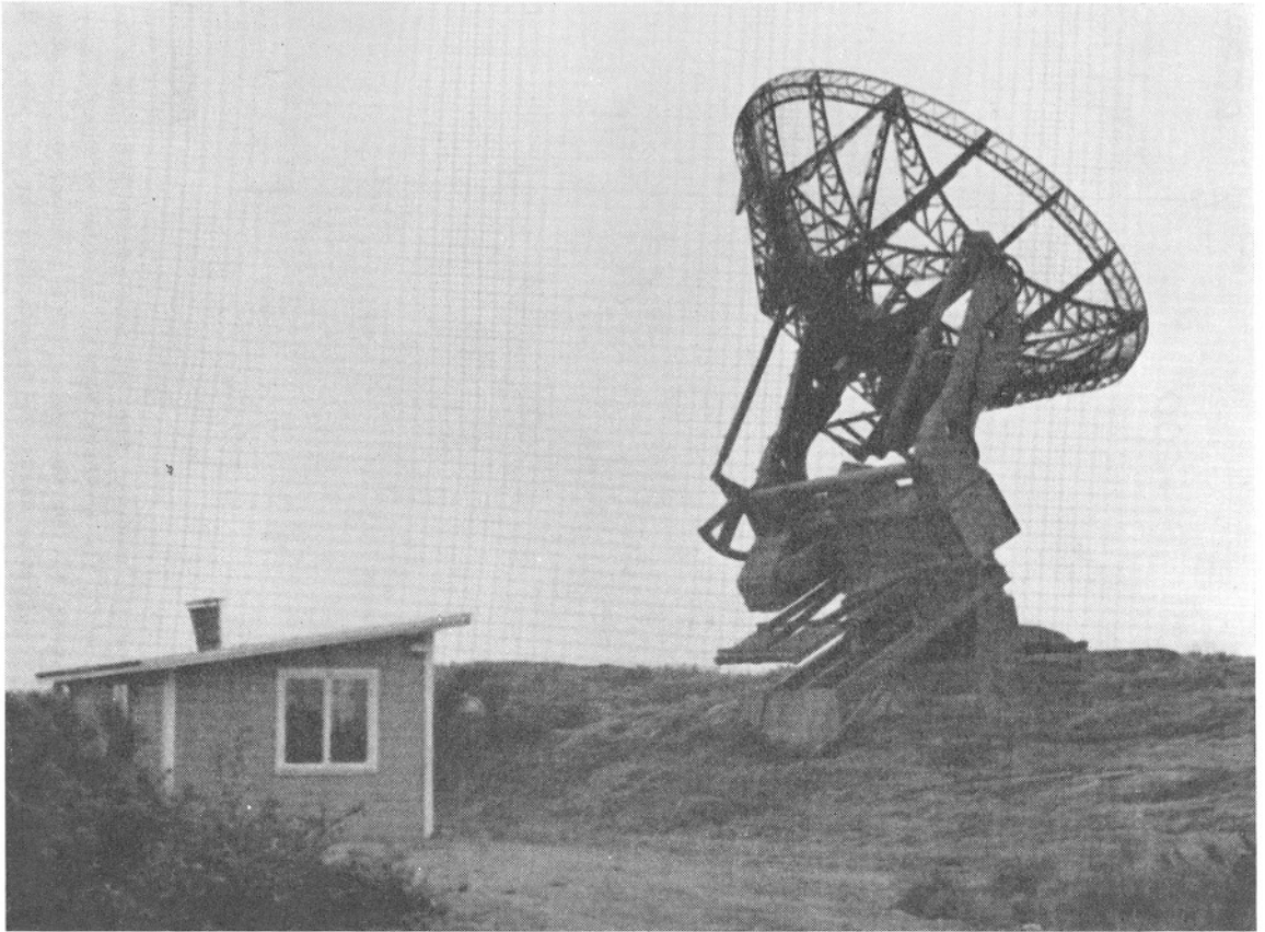
Fig. 2. A photograph of the antenna and receiver cabin. The antenna is equatorially mounted.
