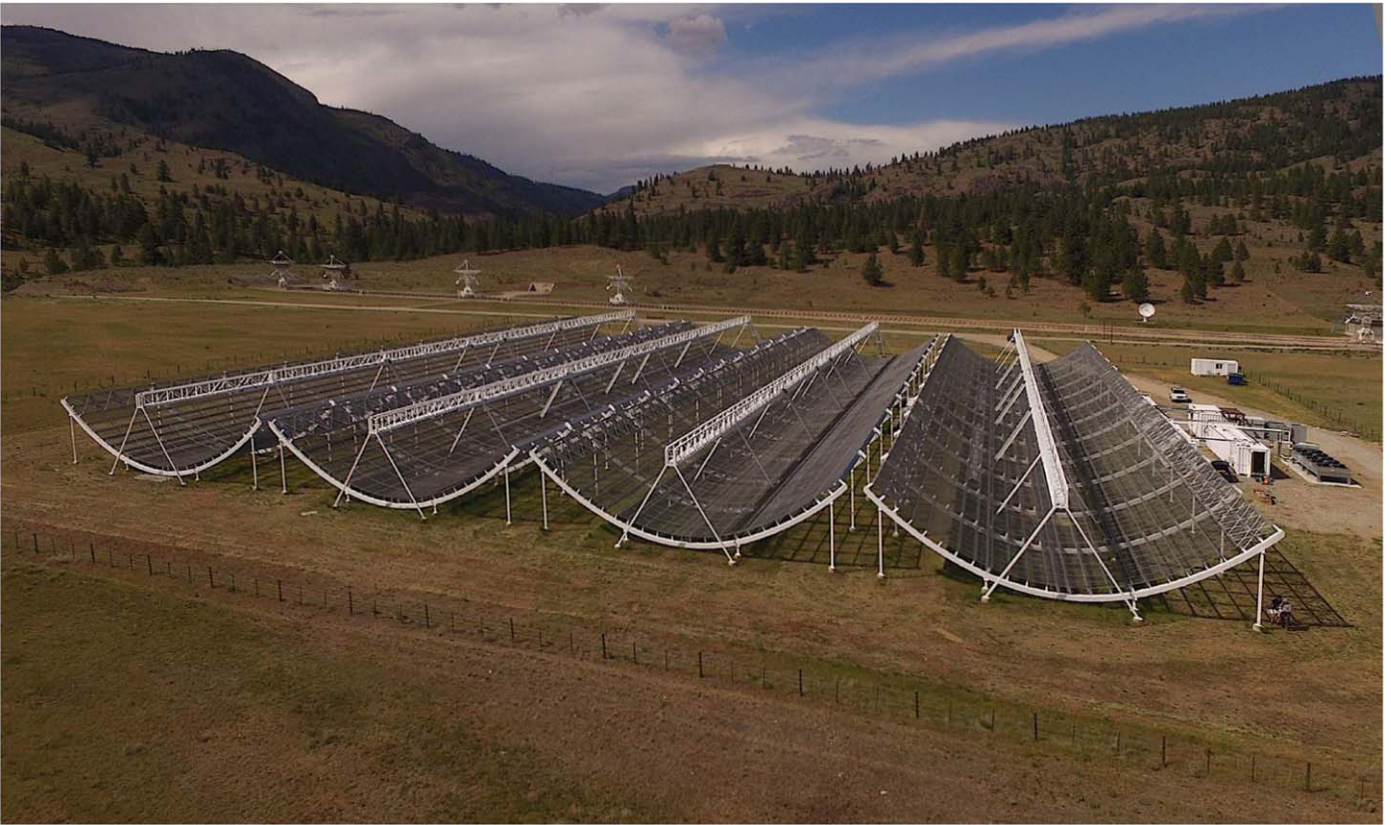
Figure 2. A photograph of CHIME looking north. The parabolic reflecting surface of each of the four cylinders is 20 m aperture, 5 m focal length, and 100 m long. The two people standing at the southeast corner (right, foreground) help to show the physical size. A total of 256 dual-polarization antennas are placed along the central 78 m of the focal line of each cylinder, beneath an 88 \text{ m} \times 0.65 \text{ m} ground plane. The focal lines are covered by and suspended from the walkways visible along each cylinder axis. Signals are amplified at each feed and brought by low-loss coaxial cables to receiver huts located in commercial RF-shielded rooms within customized RF-protective shipping containers, one located between the first and second cylinders, another between the third and fourth. After band-defining amplification, analog-to-digital conversion, a time-to-frequency transform, and half of a “corner turn,” signals are brought from the two receiver huts to additional RF-shielded rooms within the white shipping containers seen at the right, where the corner turn is completed and a spatial transform and other processing are performed. The gray and black structure at the far right is an ambient air heat exchanger associated with the water-cooling system for the X-engine in the adjacent RF-shielded rooms. Behind that, also gray, is a 0.5 MW power substation to power the instrument. CHIME is located at the Dominion Radio Astrophysical Observatory, which is protected by law and the adjacent hills from terrestrial radio interference. In the background one can see five dishes of the DRAO Synthesis telescope and a solar radio monitor.
