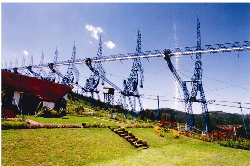
A partial view of the northern half of the cylindrical telescope after its completion. The focal line – running horizontally in the photo – with the dipoles and phase shifters can be clearly seen. The reflection of the Sun by the reflecting 'surface' can be seen as a vertical line of bright light. It is an awesome sight to see this parabolic cylinder, 530 m long, rotating about its axis as a single unit.
