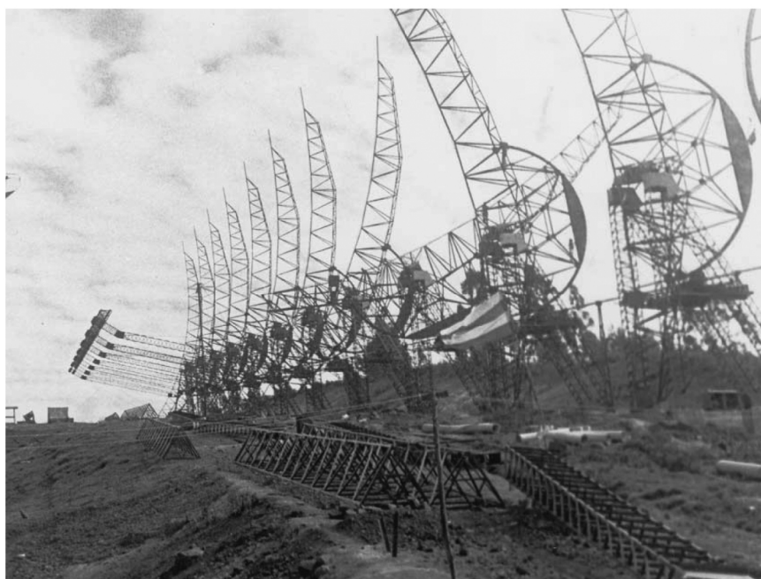
A view of the northern section of the 530 m long cylinder. The vertical frames (24 of them in all) are of parabolic shape. These support the reflecting surface, made of 1100 stainless steel wires. The horizontal structures seen on the left are supports for the 1024 dipoles and phase shifters placed along the focal line.
