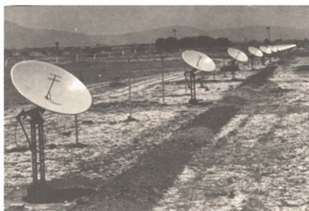
Photo on the left shows the East–West array of the 32 element radio telescope near Kalyan. This telescope, built by Christiansen for the study of the Sun, was gifted to India by CSIRO Australia. The photo on the right shows V. K. Kapahi (left) and Govind Swarup.
