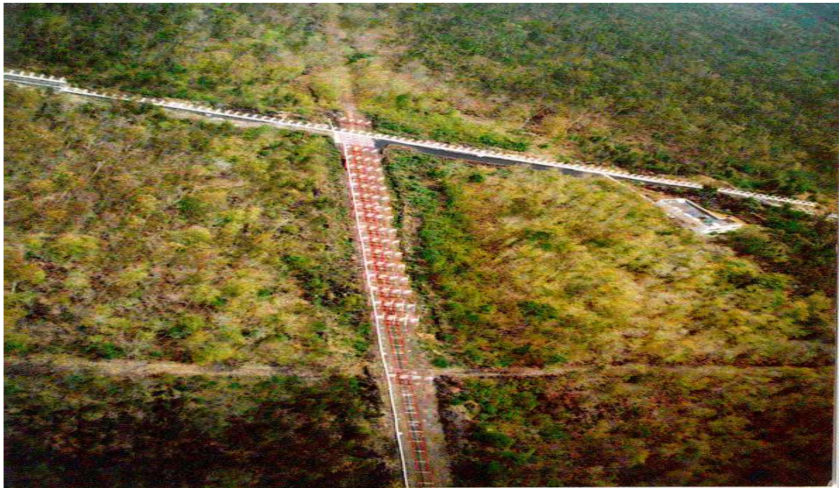
Fig. 1.5: An aerial view of the Mauritius Radio Telescope. The non-coplanarity of the EW arm can be noticed. The observatory building is also seen.
